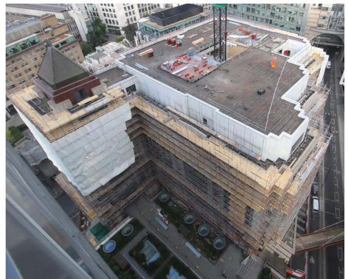
Overview Of Site Progress
